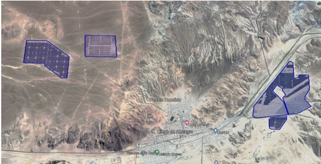
Large solar plants at 1,000m around Diego de Almagro in Chile's Atacama region
