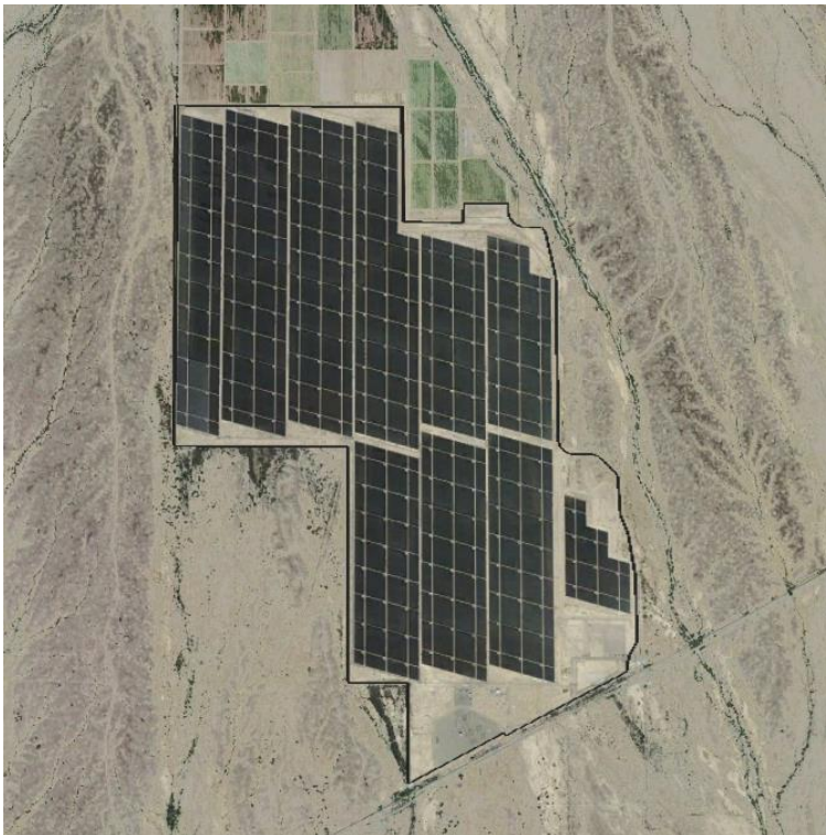
First Solar's Agua Caliente project covers 9 sq. km of semi-desert in southern Arizona. It was the world's largest individual solar plant when first commissioned in 2012
