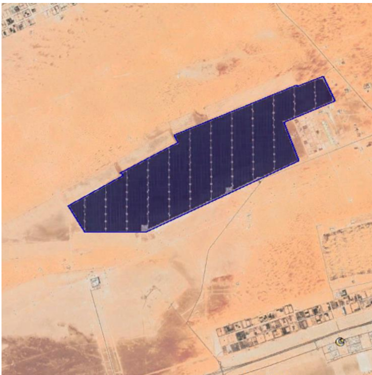
ADWEA's Sweihan plant developed with Marubeni & JinkoSolar, and built by Sterling & Wilson, densely covers 8 square km of semi-desert. It was the world's largest individual solar plant when commissioned in 2019.
